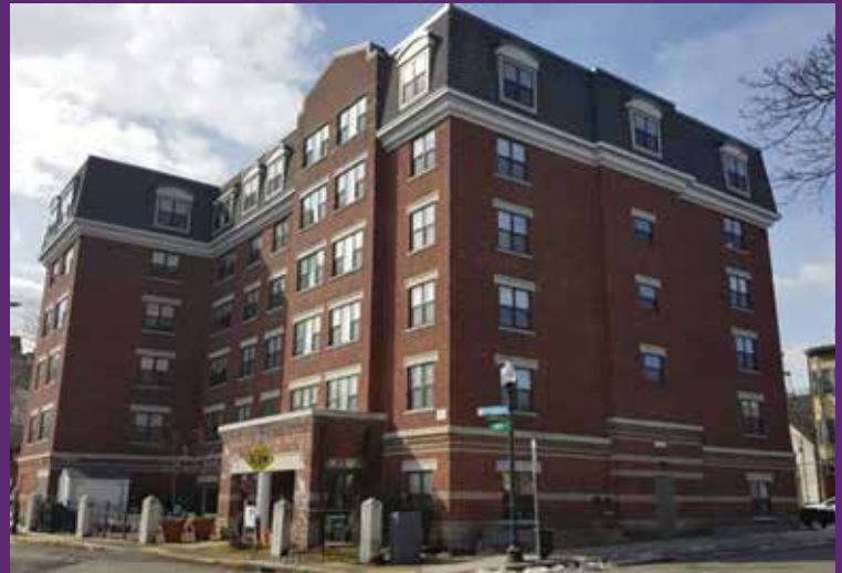
Robert A. Georgine Tower
