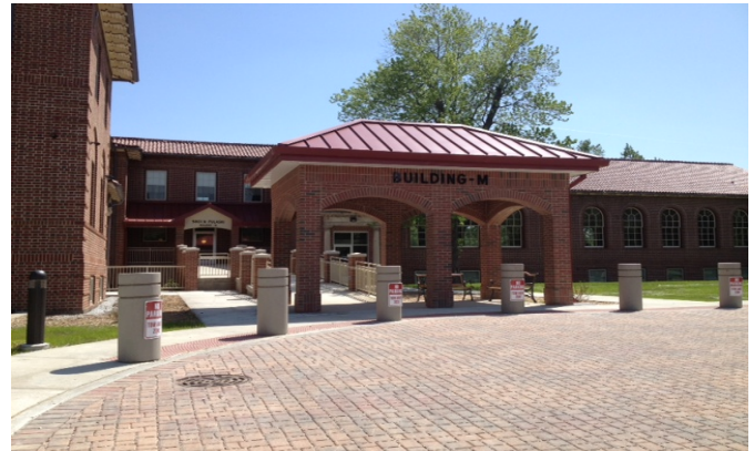
Newest Property, Edward M. Marx Apartments Chicago, IL
